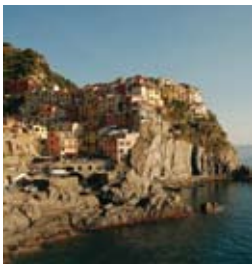
Manarola village in Cinque Terre National Park (Photo: AlterEco)
